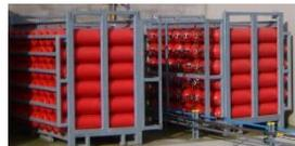
**On-site H<sub>2</sub> Storage:** Hydrogen is compressed and stored on-site, ready for fuelling.
